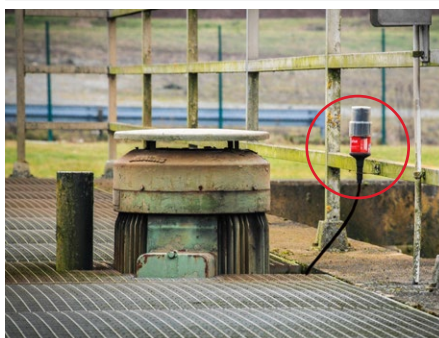
Lubrication of bearing at surface aerator
