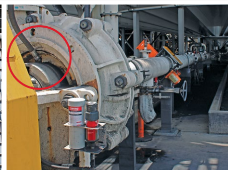
Pump bearing lubrication
