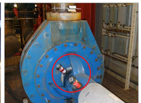
Lubrication of drive shaft on pump
