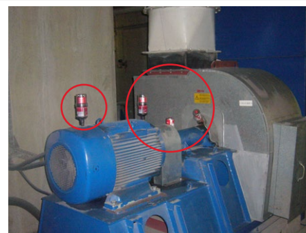
Lubrication of electric motor and shaft on secondary fan
