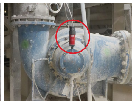
Pump bearing lubrication
