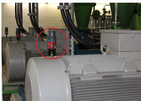
Electric motor bearing lubrication
